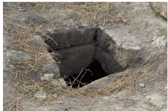
Fig. 1.100 Outer inlet of cistern (Source: BAI/GPIA).
