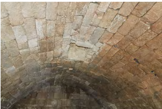
Fig. 1.99 Inner inlet of cistern (Source: BAI/GPIA).
