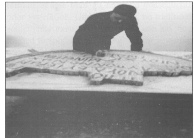
25. The fabric removed after being wetted first with water and then with a substance known as Americana. A heavy, flatted, rectangular piece of iron measuring 12 x 17 cm, with an upper handle, was used to press the tesserae into the new mortar; thereby encouraging the mortar to penetrate between them.
