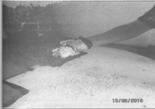
20. The surface of the fibreglass was then roughened using epoxy and beads in order to provide grip for the mortar.
