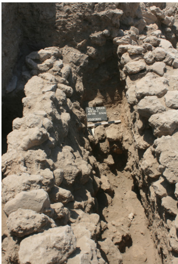
Fig. 1.16 The Early Bronze Age city wall's construction, Stratum 25, Area I, Square AO 115, Complex A, Contexts (from left to right) 6463, 6509, and 6464 (Source: BAI/GPIA).
